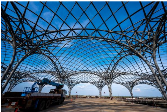
Figure 5 A new Phnom Penh Airport under construction on Nov. 9, 2022. Photo: Xinhua
